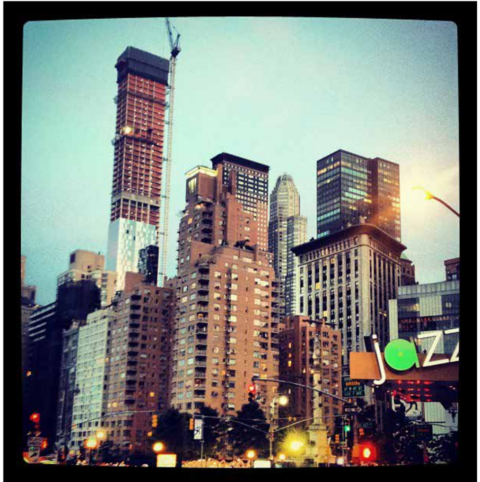
One57, dubbed the “Billionaires Haven,” under construction in July, 2012.
