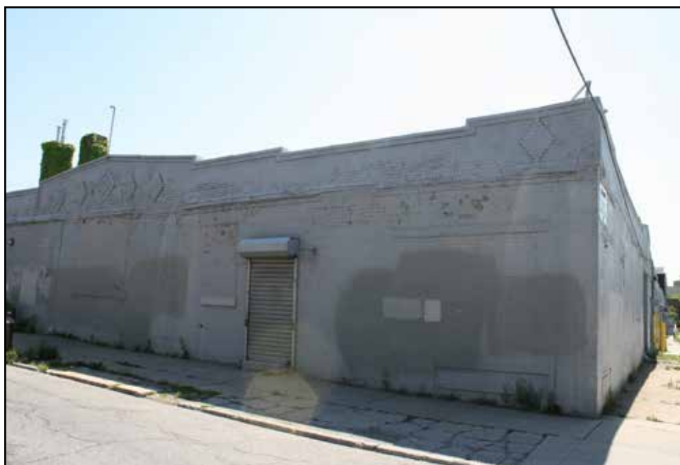
The exterior walls of 363 Bond Street
